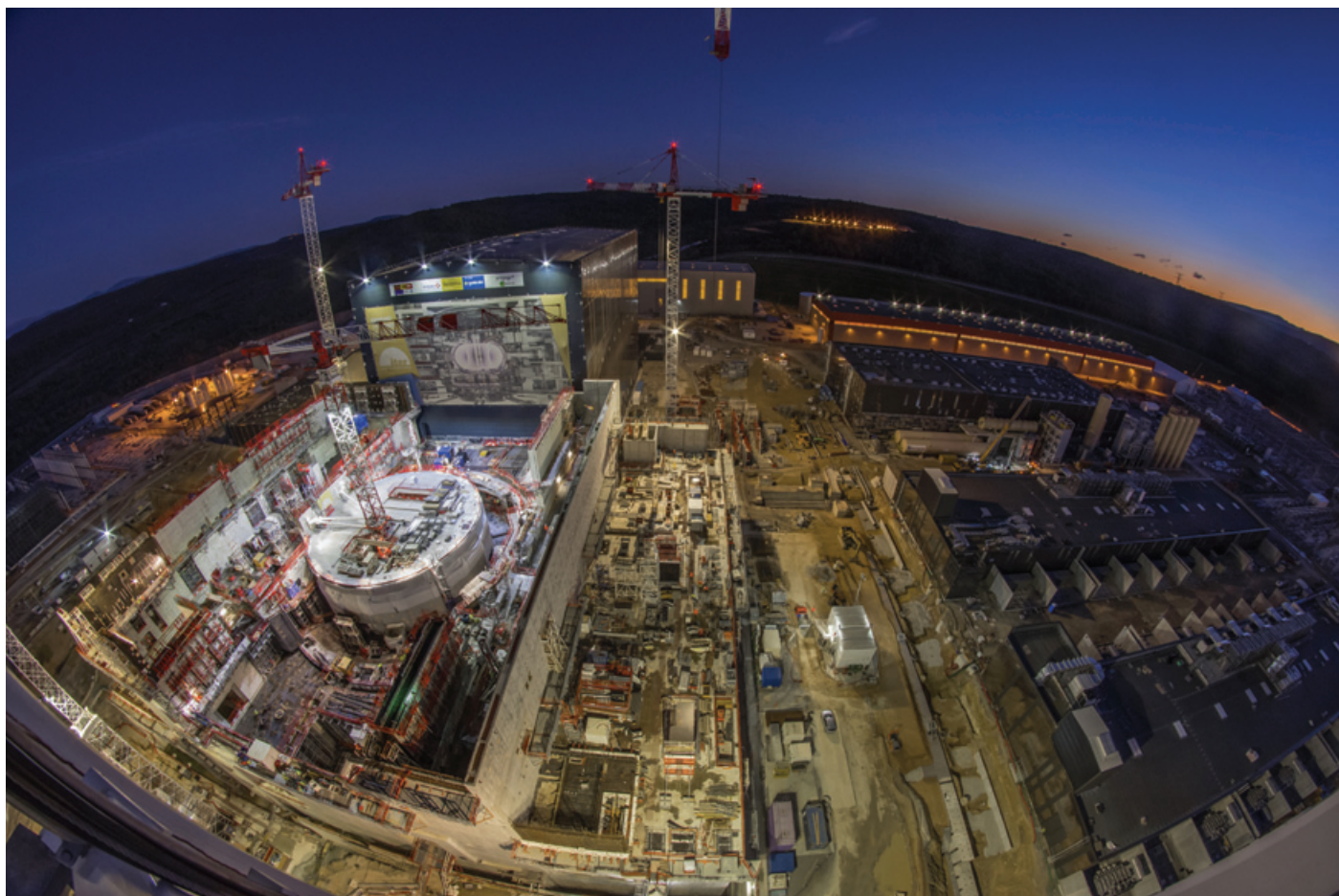
The heart of the ITER installation: to the left, the Tokamak Complex with the circular structure of the "bioshield", a 3-meter-thick steel-and-concrete cylinder that will enclose the ITER Tokamak; to the right, the installation's industrial facilities (power conversion buildings, cryoplant, winding facility, etc.) (December 2018). © ITER Organization.
