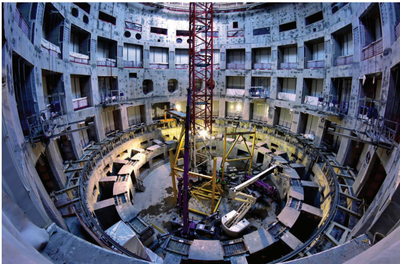
The 23,000-tonne ITER Tokamak will rest on a massive circular “crown” at the bottom of the bioshield. The openings in the cylindrical structure are for the different systems that need to reach into the machine: power feeders, vacuum pumping, heating, cryogenics, cooling water, diagnostics, etc. © ITER Organization.
