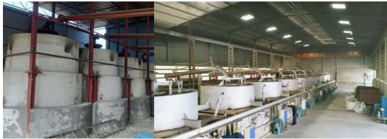
Dry Distillation Still reactor
