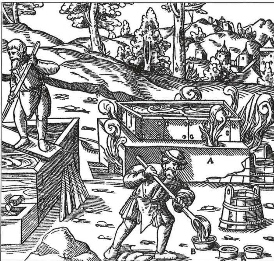
Chaudière (A), moules (B), gâteaux (C).
