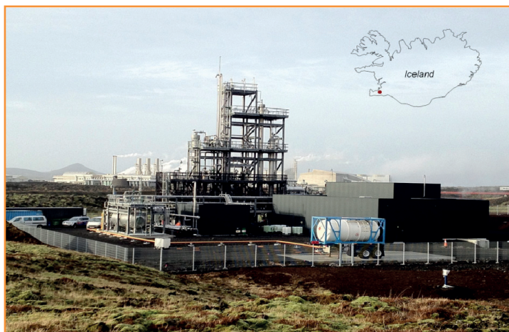
Figure 2 - The "George Olah carbon dioxide to renewable methanol plant" of Carbon Recycling International in Iceland based on local geothermal energy: the first commercial carbon dioxide recycling plant operating in the world. Courtesy: K.C. Tran, CEO, Carbon Recycling International, Iceland.
