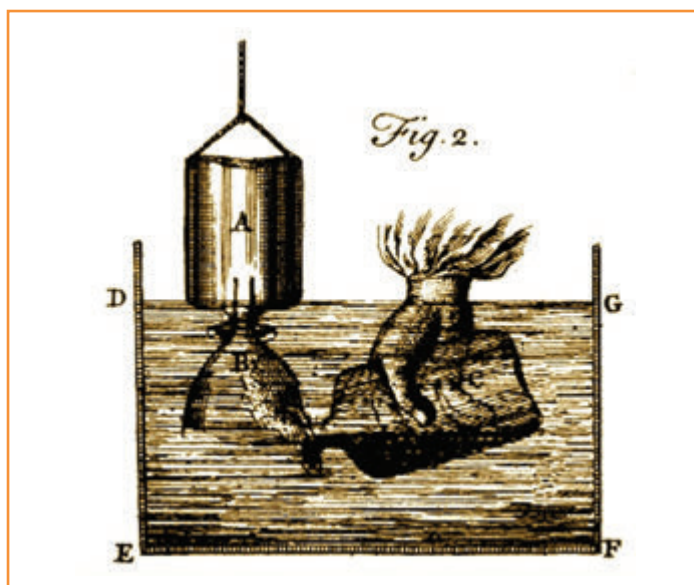
Figure 4 - Cavendish's device for transferring gases. From Philosophical Transactions (1766), vol. 56, plate 7, p. 141.
