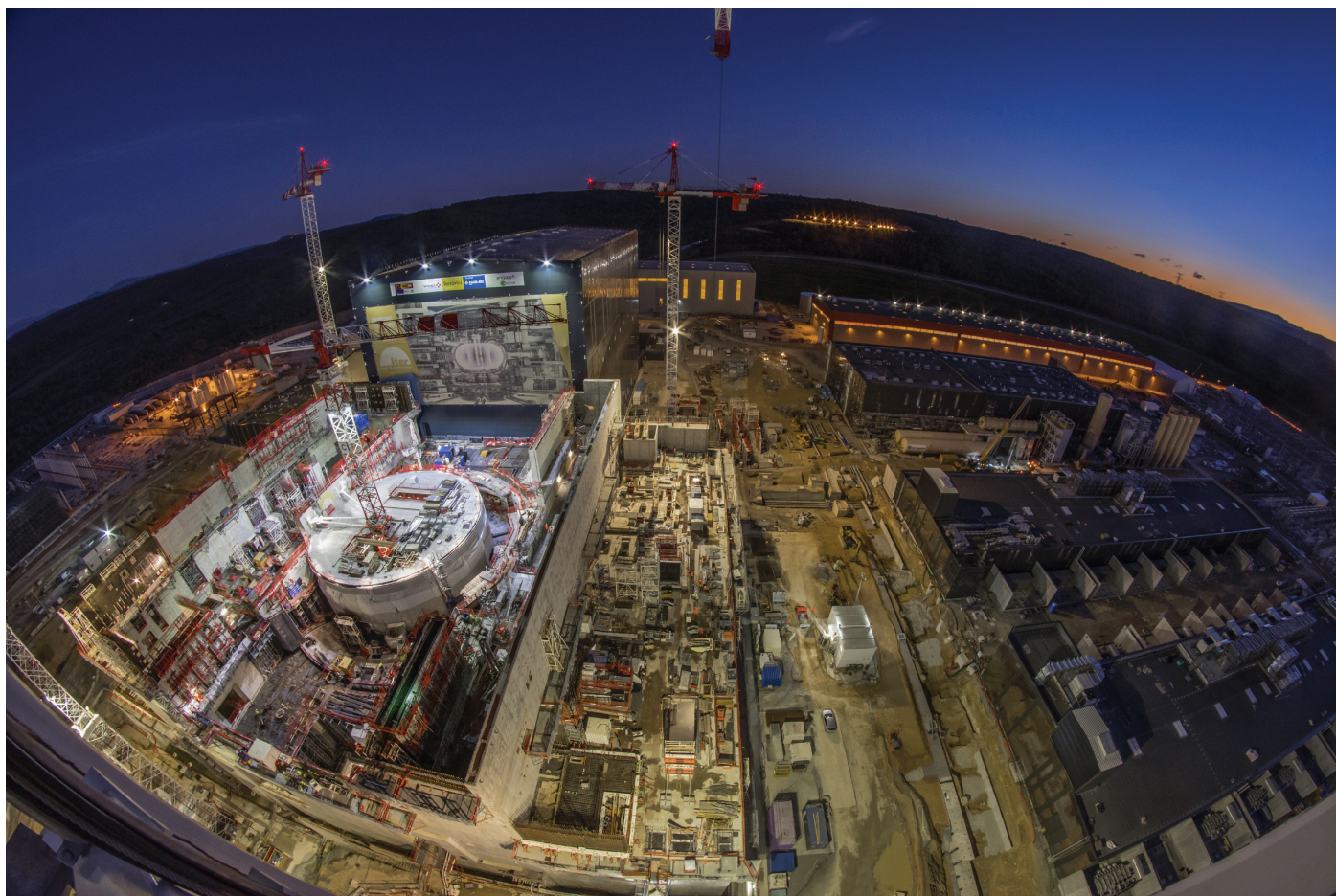
The heart of the ITER installation: to the left, the Tokamak Complex with the circular structure of the "bioshield", a 3-meter-thick steel-and-concrete cylinder that will enclose the ITER Tokamak; to the right, the installation's industrial facilities (power conversion buildings, cryoplat, winding facility, etc.) (December 2018). © ITER Organization.
