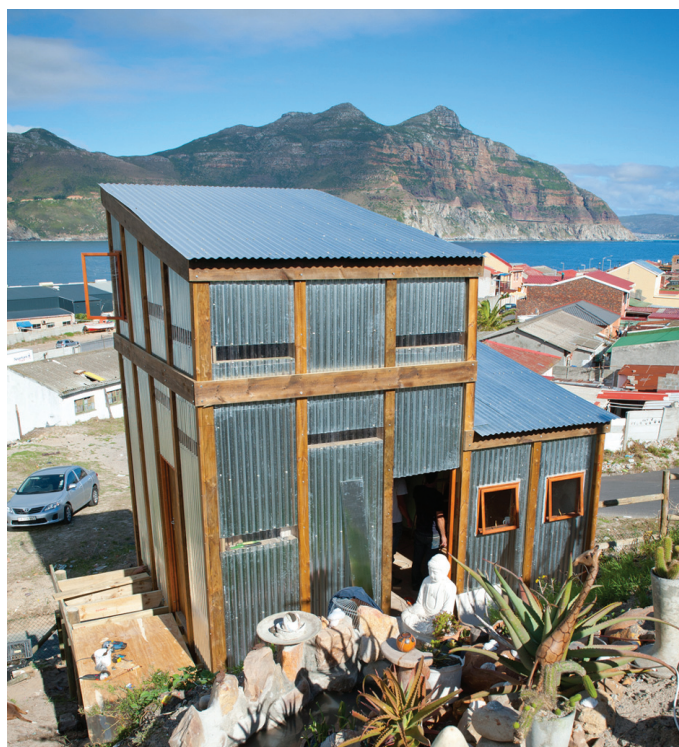
The Light House in Hout Bay (Cape Town, South Africa) built by designers and builders Stephen Lamb and Andrew Lord ( www.visi.co.za/this-is-the-house-that-xoma-wanted ). Photo: Stephen Lamb.
